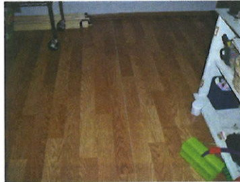
Photo 6 – North/south-oriented 18/32" separation of the flooring in the Unit A dining room, located 3' south of the opening to the hallway.
