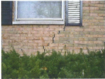
Photo 3 – Vertical and horizontal 16/32" (bottom of window) to 20/32" (top of Unit A window) mortar joint step crack in the brick veneer at the north window on the west elevation.
