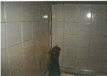
Photo 5 – Vertical 8/32" crack and separation in the tile grout on the south wall of the Unit B kitchen on the east side of the built-in stove.
