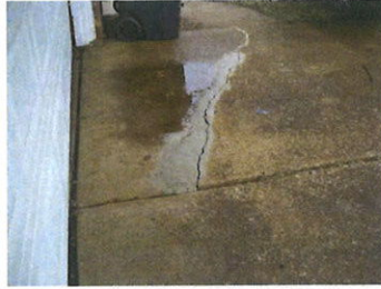
Photo 4 – Previously patched and reopened diagonal 8/32" crack in the east driveway slab adjacent to the garage overhead door on the south elevation of the structure.
